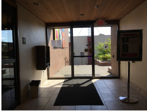
(Photo 59) Non-compliant toe kick @ egress door
