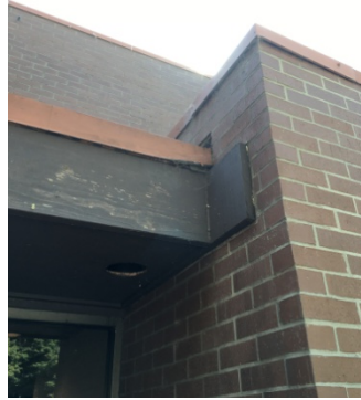
(Photo 60) Weathering & water damage
