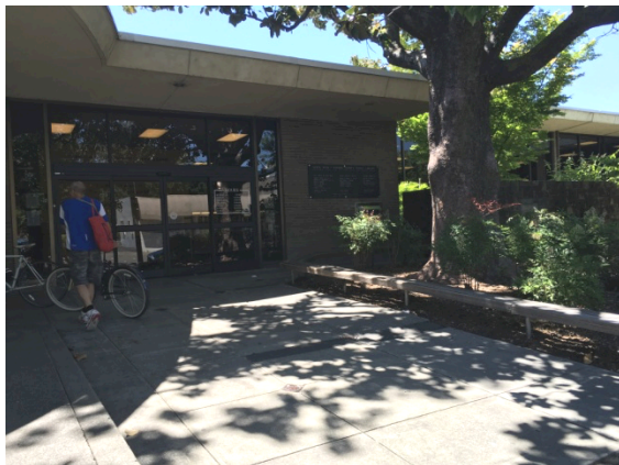
(Photo 02) Sloped Walkway @ Main Entrance
