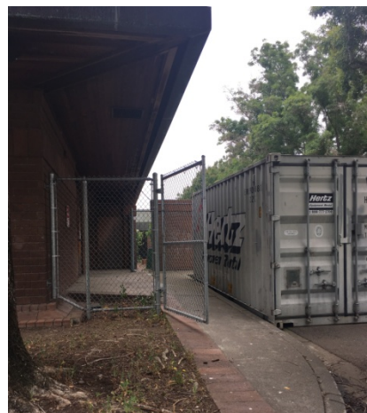
(Photo 43) Gated, chain-link construction fence
