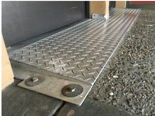
(Photo 24) Modified threshold
