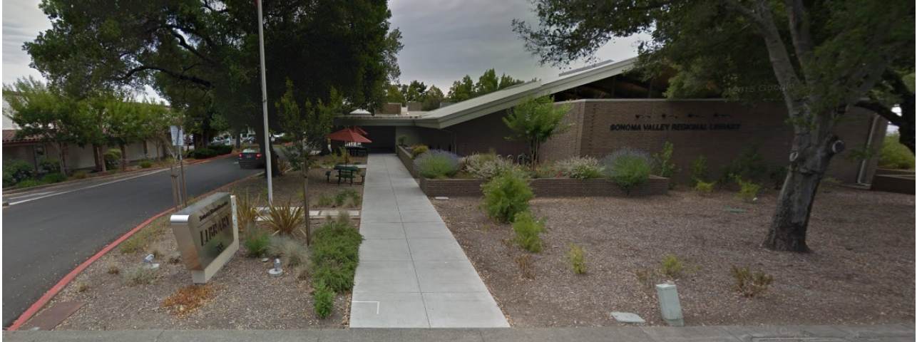
(Photo 34) Main Entrance - 755 W. Napa Street Image Courtesy of Google
