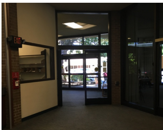
(Photo 04) Main Exit/Egress Door @ Lobby
