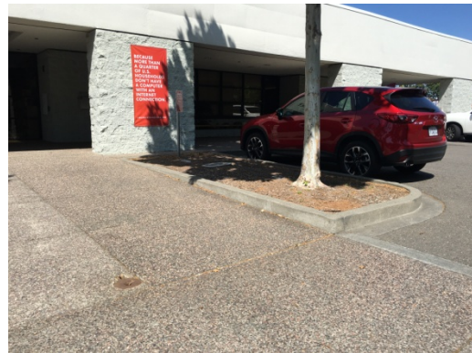
(Photo 68) Non-compliant path of travel
