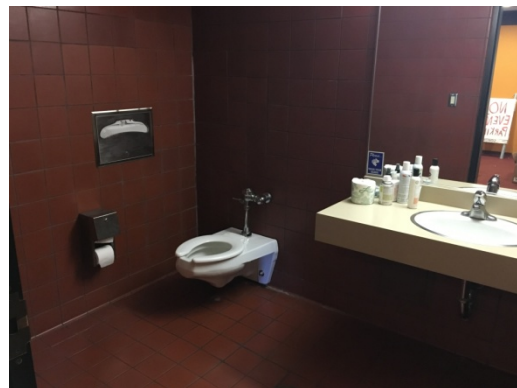
(Photo 80) Non-compliant staff restroom
