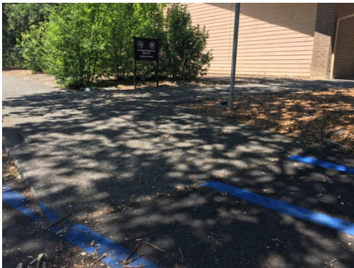
(Photo 82) Non-compliant path of travel
