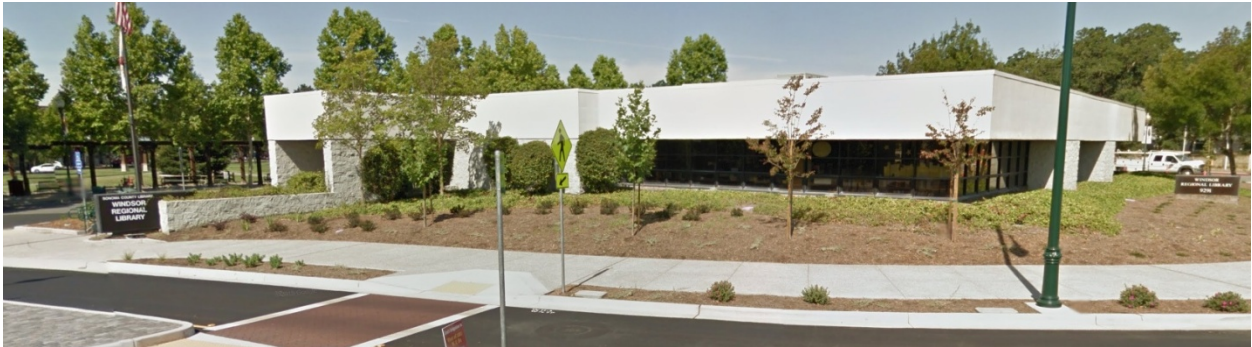
(Photo 66) 9291 Old Redwood Highway Image Courtesy of Google
